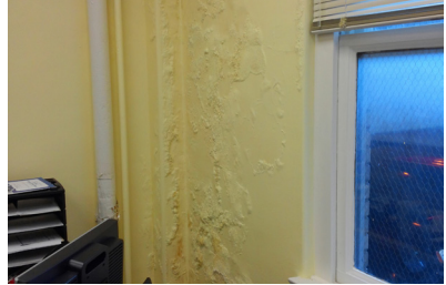
Interior Entire Area Example
