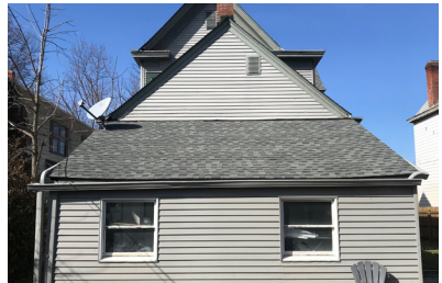
Exterior Entire Area Example
